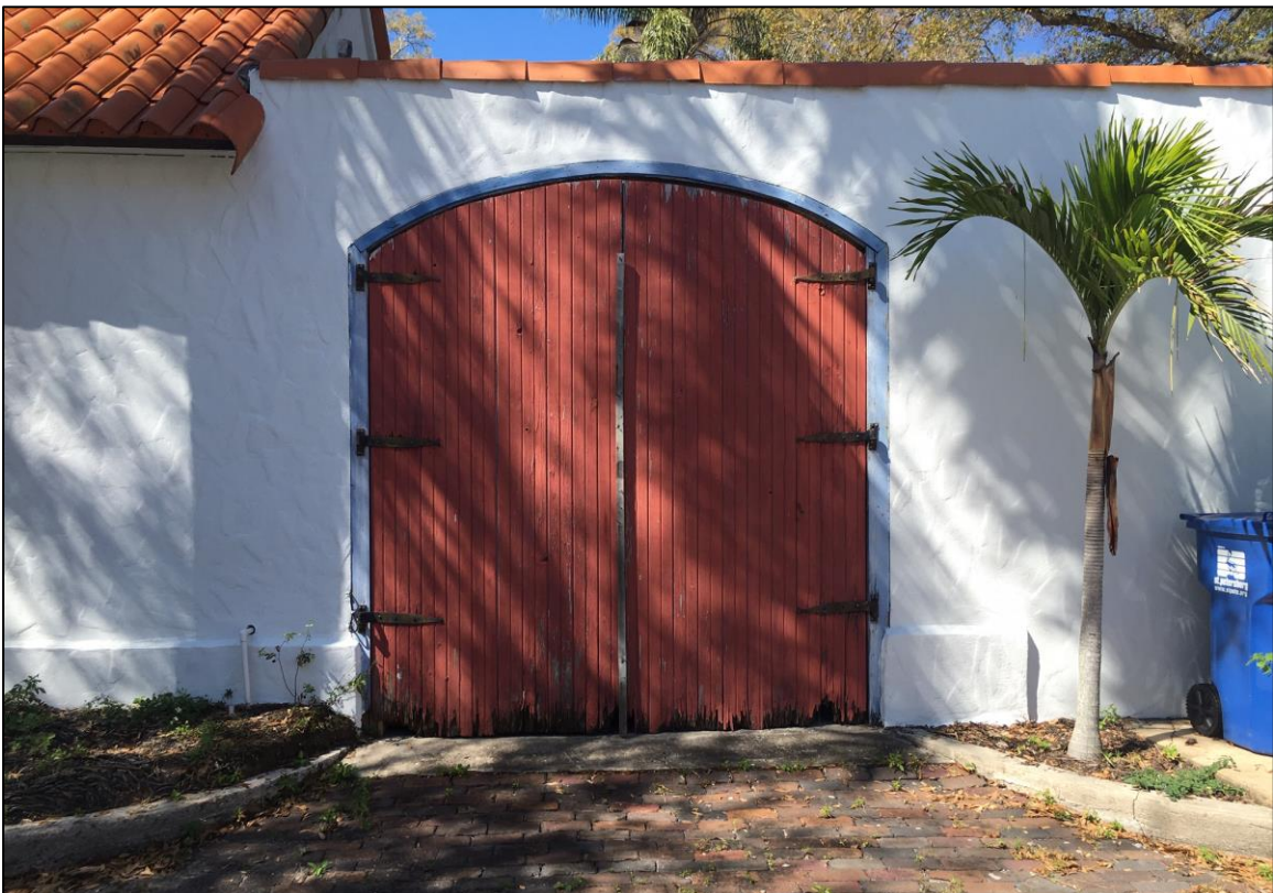
Figure 3: Close up photograph of the existing garage door.
